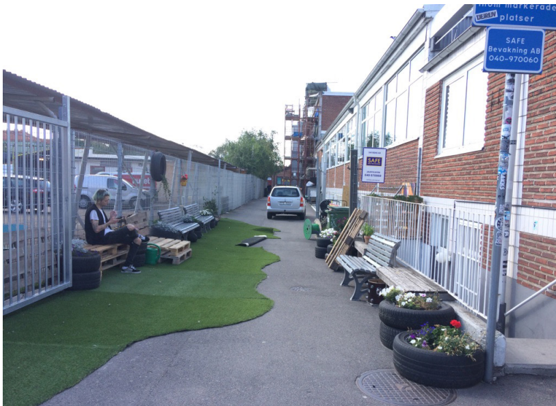
Figure 4.7. Entrance to the basement where Plan B was located before 2017. Photograph by the author
